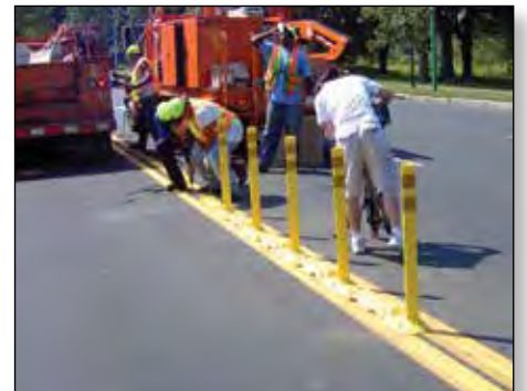
Installing Interstate Grade Curb
