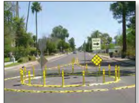
Phoenix AZ traffic calming circle
