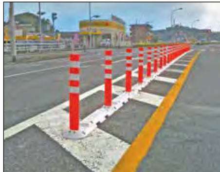
Miyazaki National Highway
