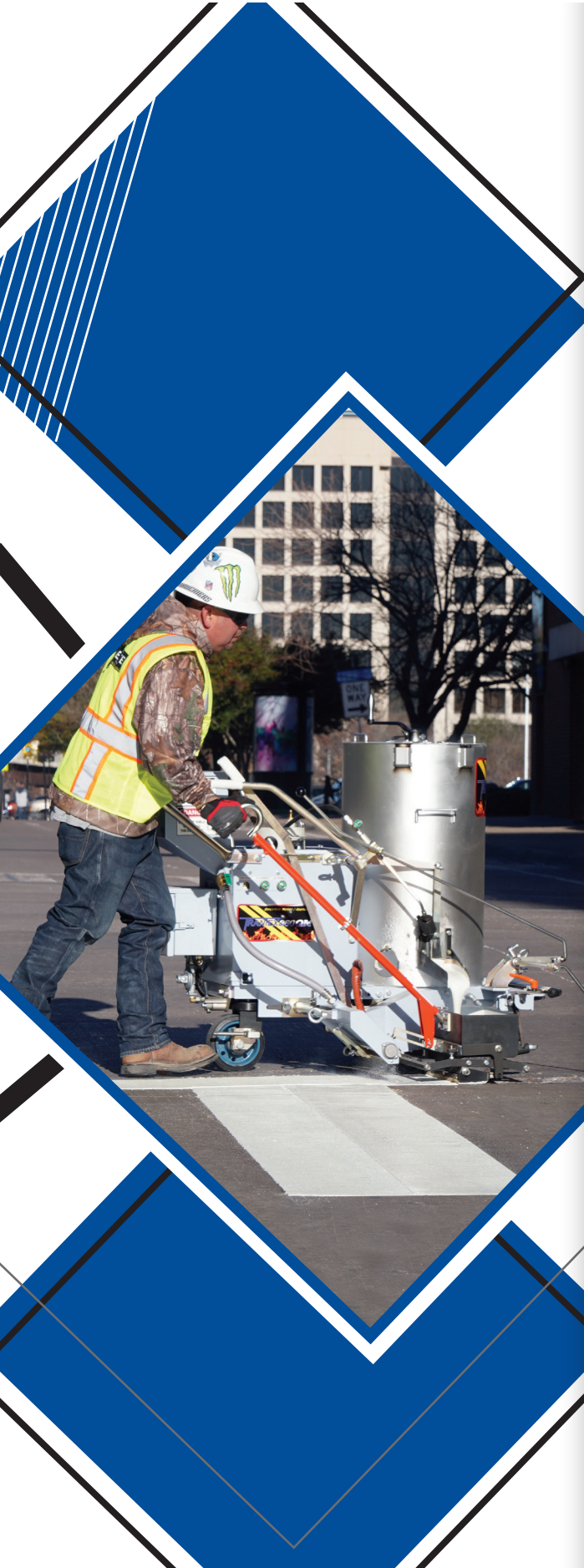
Positive direct-drive bead dispense — no frictional wheels
