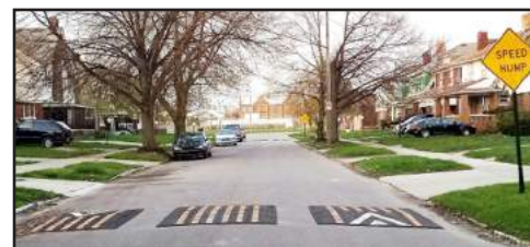
Cushions should be placed in a series with distances of 200 to 500 feet between sets.
